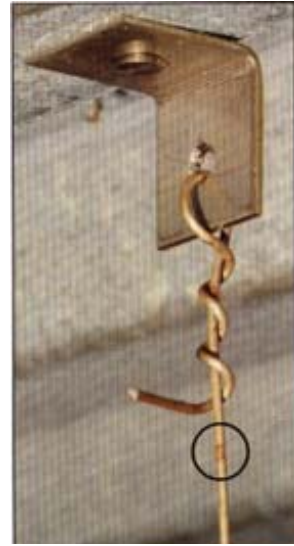
Suspended ceiling support wire (SCC ringed)
