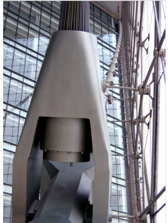
Figure 7: View of cast steel rocker with stainless steel cables (Photo: Skidmore, Owings & Merrill LLP)
