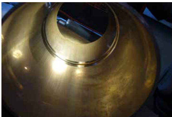
Finished weld showing root penetration on pipe bore (Courtesy Eucaro Buntmetall GmbH)
