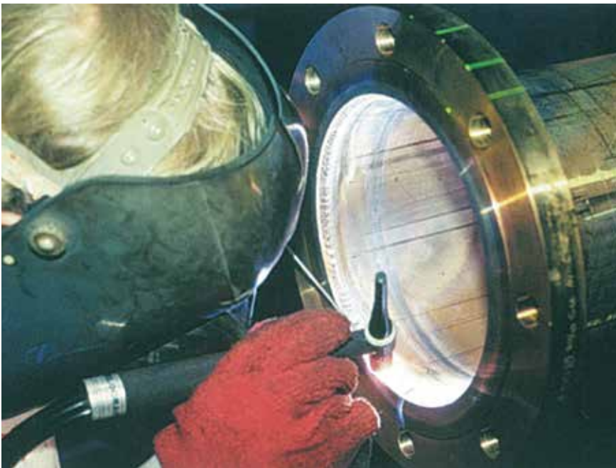
TIG (GTAW) welding a 90-10 copper-nickel assembly
