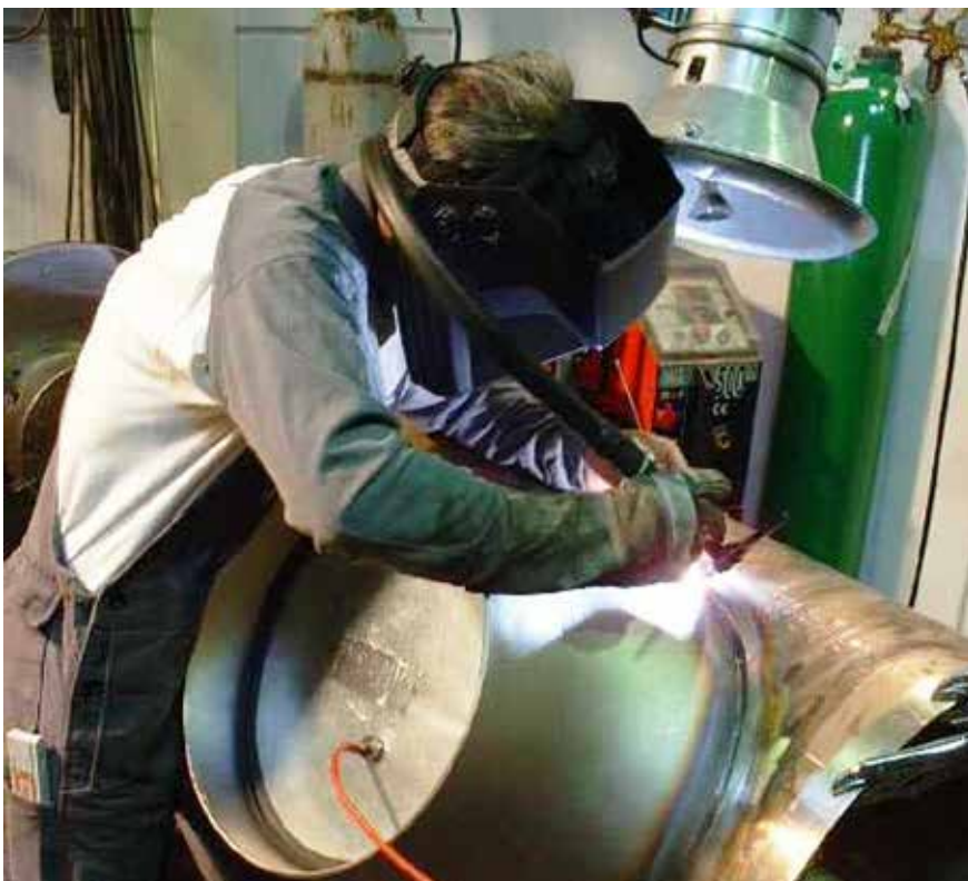
TIG (GTAW) welding 90-10 copper-nickel assembly. Note baffle for backing gas supply at root run stage (Courtesy Eucaro Buntmetall GmbH)
