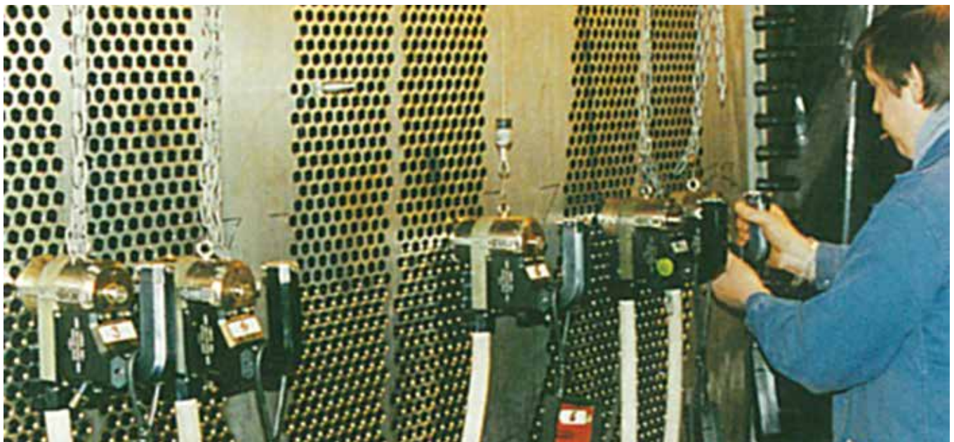
Tube to tubesheet welding of a large heat exchanger using automatic TIG (GTAW) welding heads (Courtesy Arc Machines Inc)
