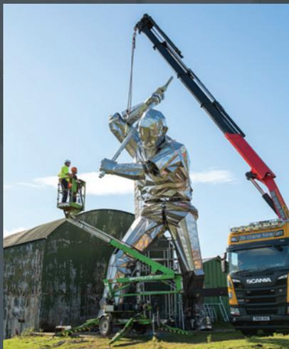
*John McKenna at the test build. The figures were made in sections in the studio and assembled outdoors with the aid of cranes and elevators.*
