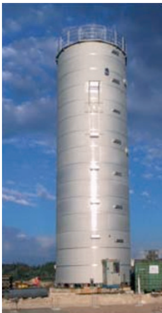
Figure 10 LDX 2101 (S32101) duplex stainless steel fermentation tank for the production of ethanol. (Courtesy of Outokumpu)
